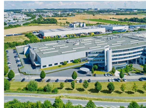
Innovation Center Power Reliability Paderborn | Germany
